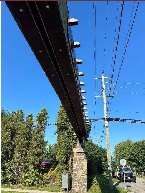
Figure 3: Underside of North Gate Looking West
