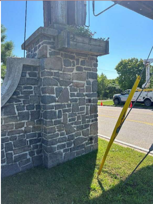
Figure 15: West Face of North Support - East Gate
