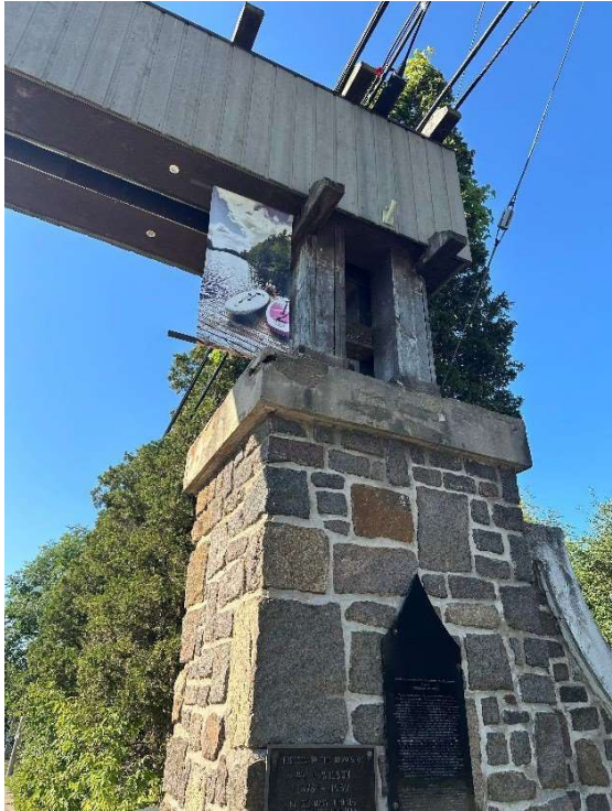
Figure 7: Concrete Cap on Masonry Support - North West
