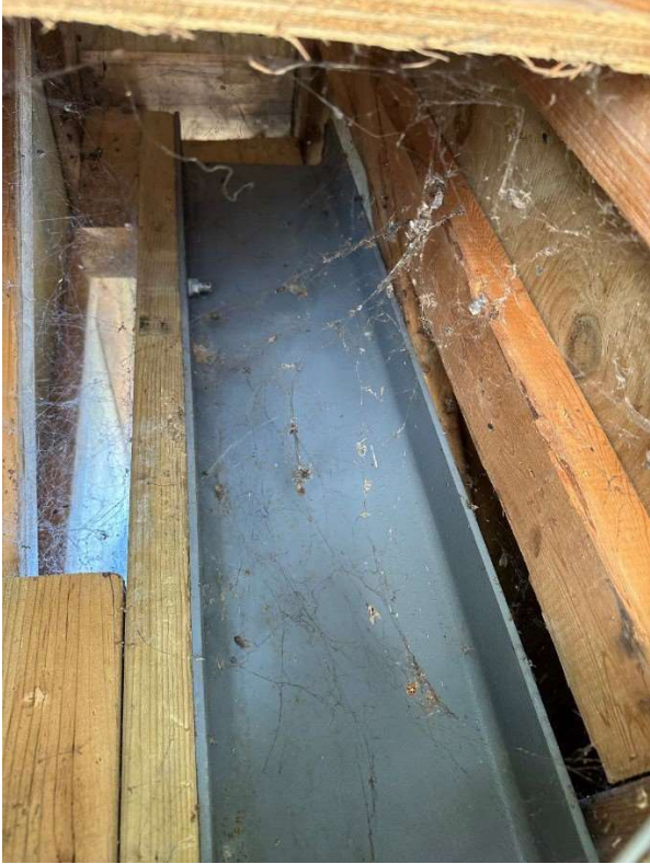
Figure 21: Structural steel in good condition - East Gate
