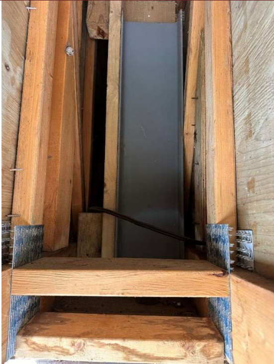
Figure 27: Wood and Steel in good condition - West gate North Side
