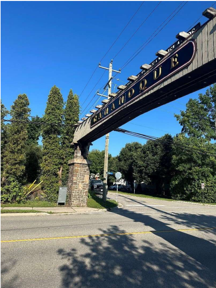
Figure 1: North Gate Looking South
