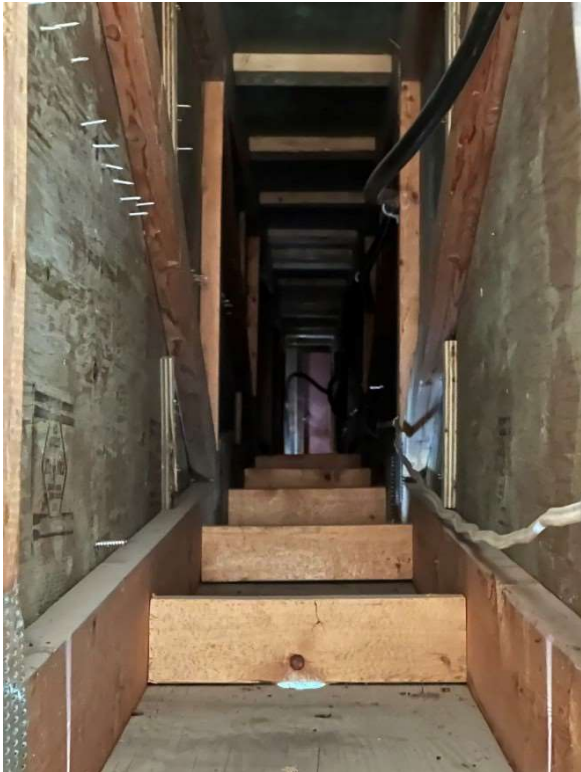
Figure 12:Inside of North Gate North Arch
