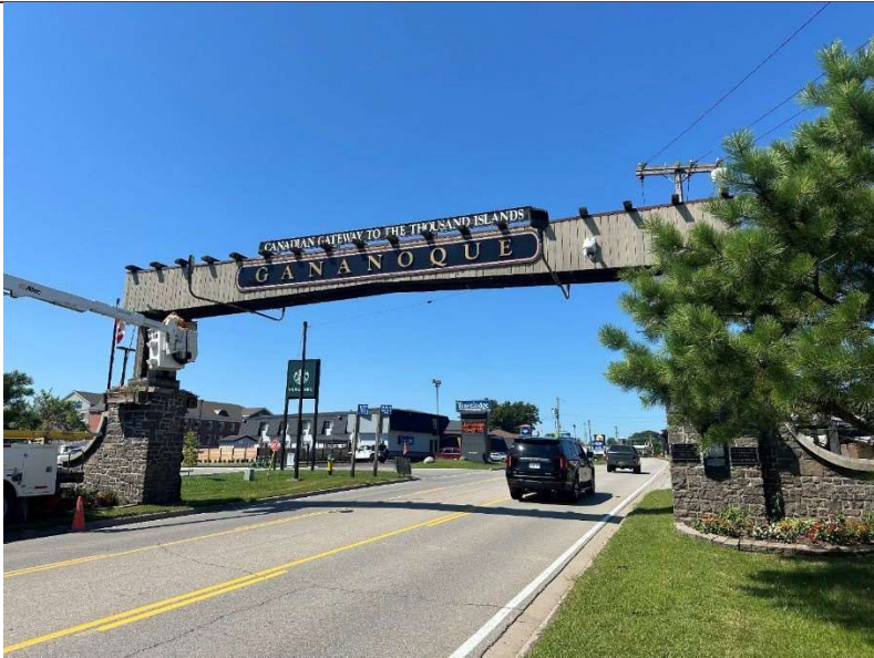
Figure 13: East Gate Looking West
