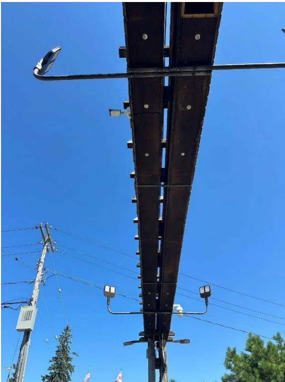
Figure 18: Underside of East Gate
