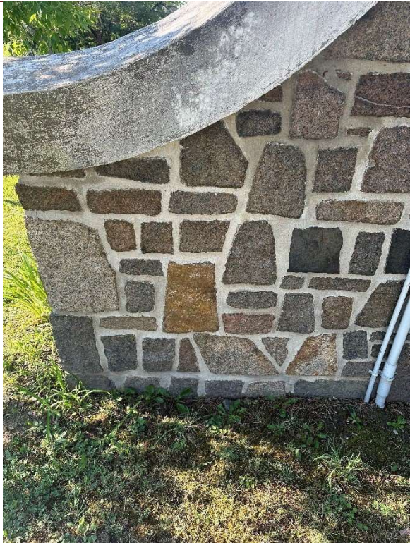
Figure 5:Wing Wall at North Gate
