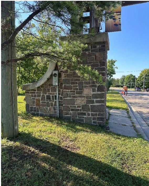
Figure 4: NE Masonry Support
