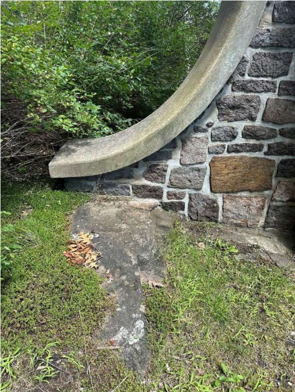
Figure 26:North Support Looking East - West Gate
