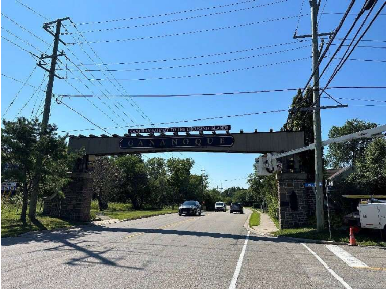
Figure 2: North Gate Looking North
