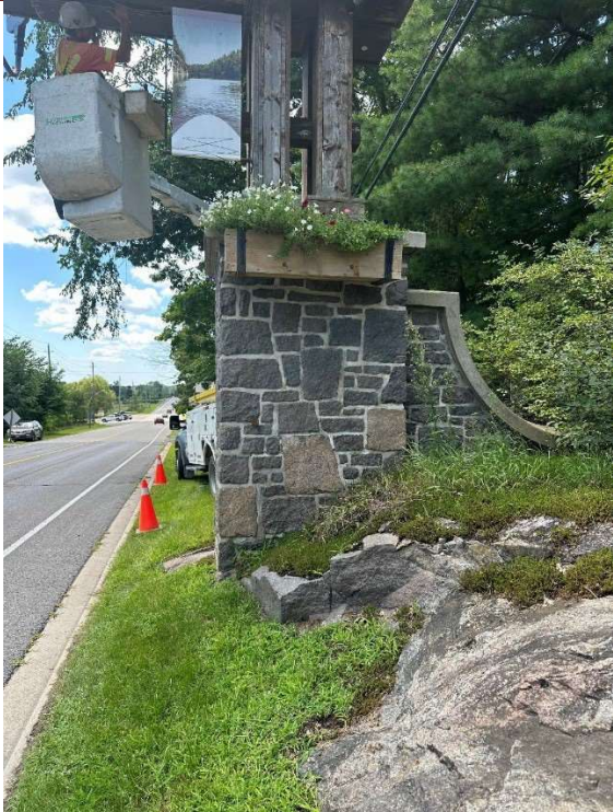
Figure 25:North Support Looking West - West Gate
